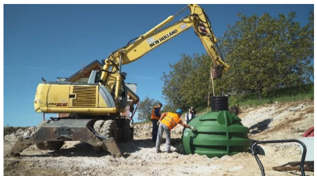
Picture 3: Installing the tank
