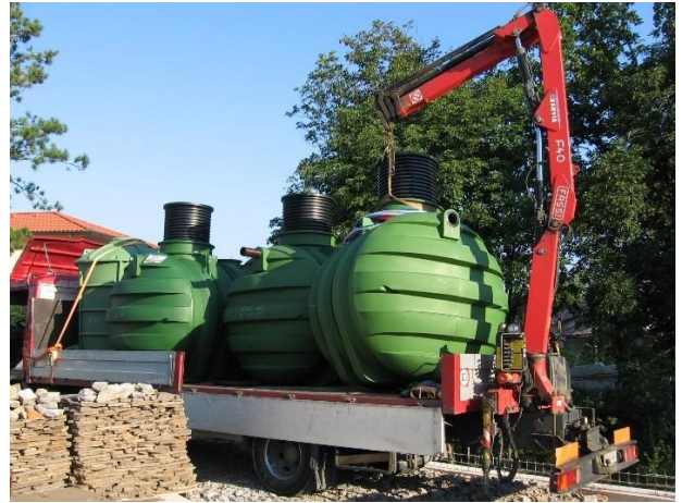
Picture 1: Correct transportation and unloading
