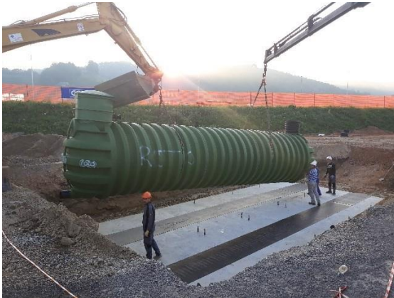
Picture 4: Installing the tank
