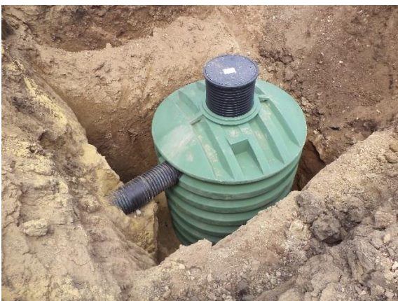
Picture 6: Installed tank
