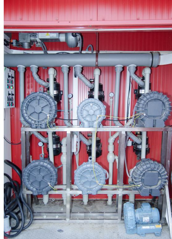
*At the back of the control room are all the blowers that supply air to the tanks*
