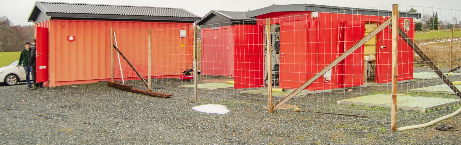
The entire facility, on the right operating building with blowing machines (open door on the left) and control room (open door on the right) behind to the left chemical container and behind to the right sludge dewatering. All process tanks are fenced off.
