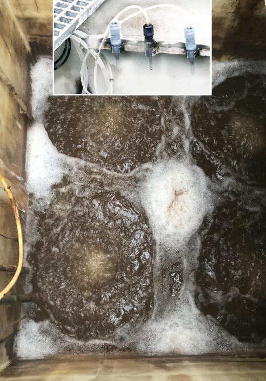
*From the equalization tanks - inset image at top shows dosing of pix, adblue and sulfuric acid*
