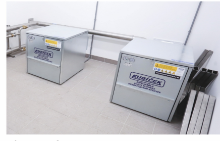
Blowers for aeration
