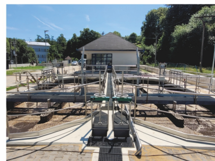
Opened construction solution
