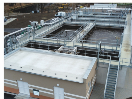
Opened construction solution
