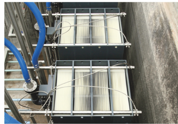
Installation of membrane modules
