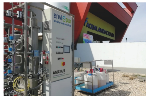
Pilot-scale testing at Aqualand Moravia (CZ)
